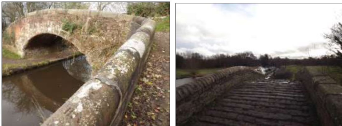
Figure 6: Turnover bridge No.100 at Meaford; Brick paved surface of bridge No.109 at Great Haywood.
