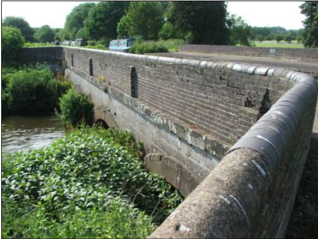
Figure 67 : Early Brindley aqueduct over the Trent at Haywood junction.
