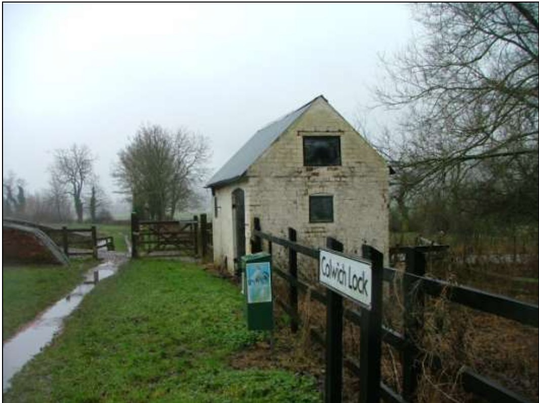
Figure 77: Maintenance building opposite Colwich Lock House
