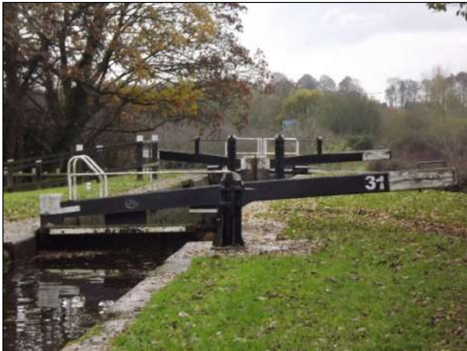
Figure 2: Typical narrow lock with single top gate and double bottom gates
