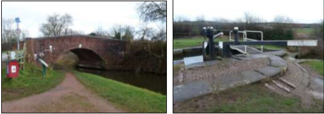
Figure 34: Aston Bridge and Aston Lock with preserved historic paving surfaces
