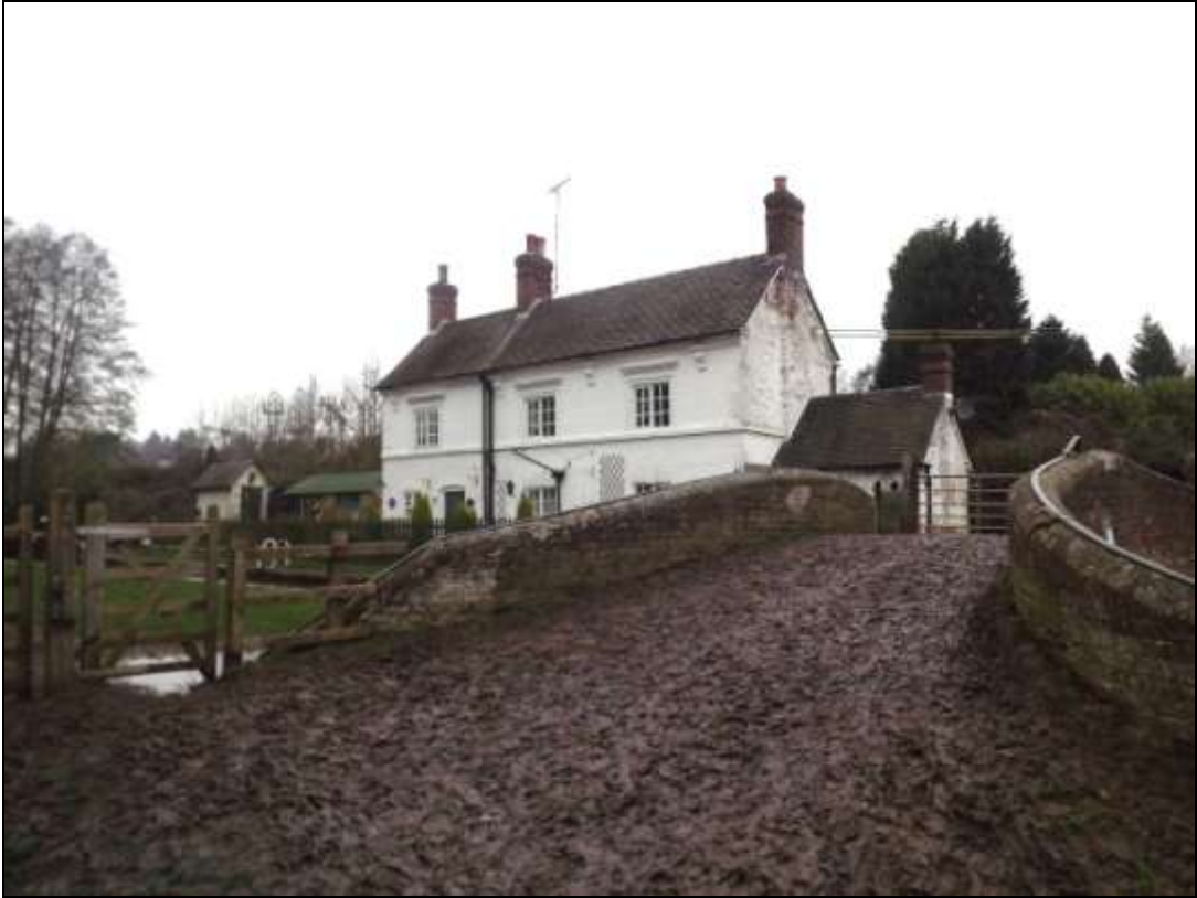
Figure 14 Grade II listed Colwich Lock Cottage with elaborate window decoration, single storey office and listed privy to the left over canal culvert.
