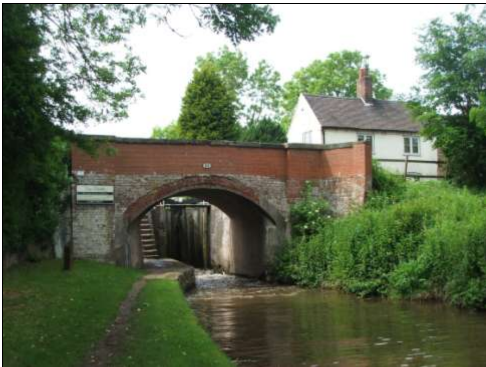
Figure 44: Sandon Bridge with rebuilt parapet and lock keepers cottage behind
