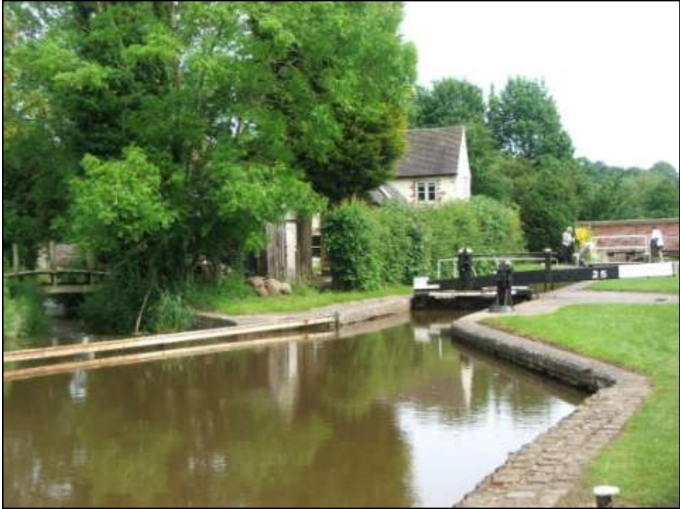
Figure 45: Sandon lock, weir, lock cottage and bridge.
