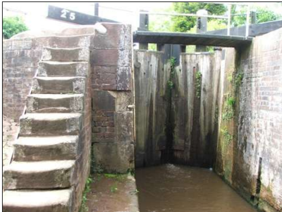
Figure 3: Oak lock gates, footbridge and stone steps at Sandon Lock.
