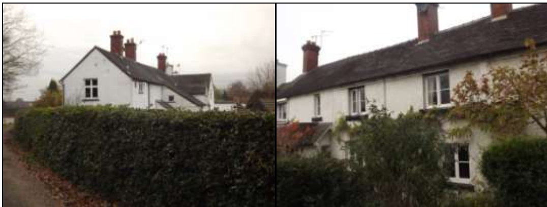
Figure 16 1 and 2 Canal Side
