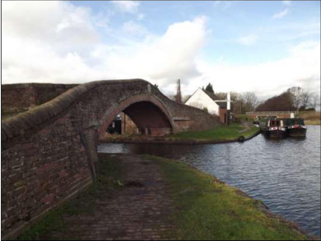
Figure 8 bridge 109 at Haywood Junction
