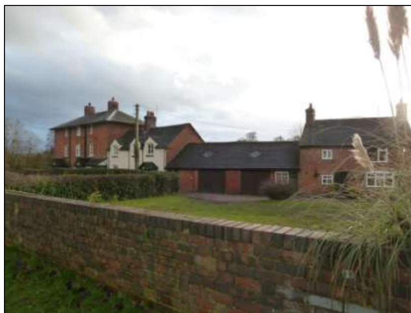
Figure 42: Sandon Lock mill, cottages and former smithy
