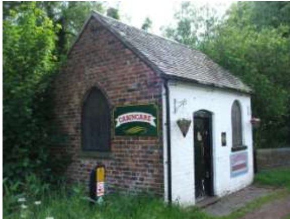
Figure 10: Banksman's cottage at Haywood Junction
