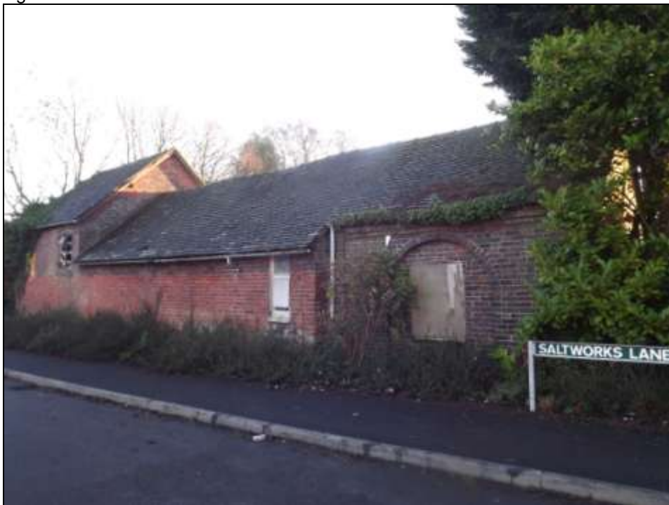
Figure 56: Redundant former agricultural buildings at Salt Works Farm
