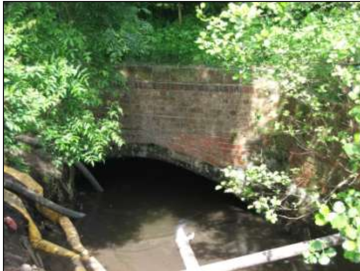
Figure 7: Brick culvert at Weston
