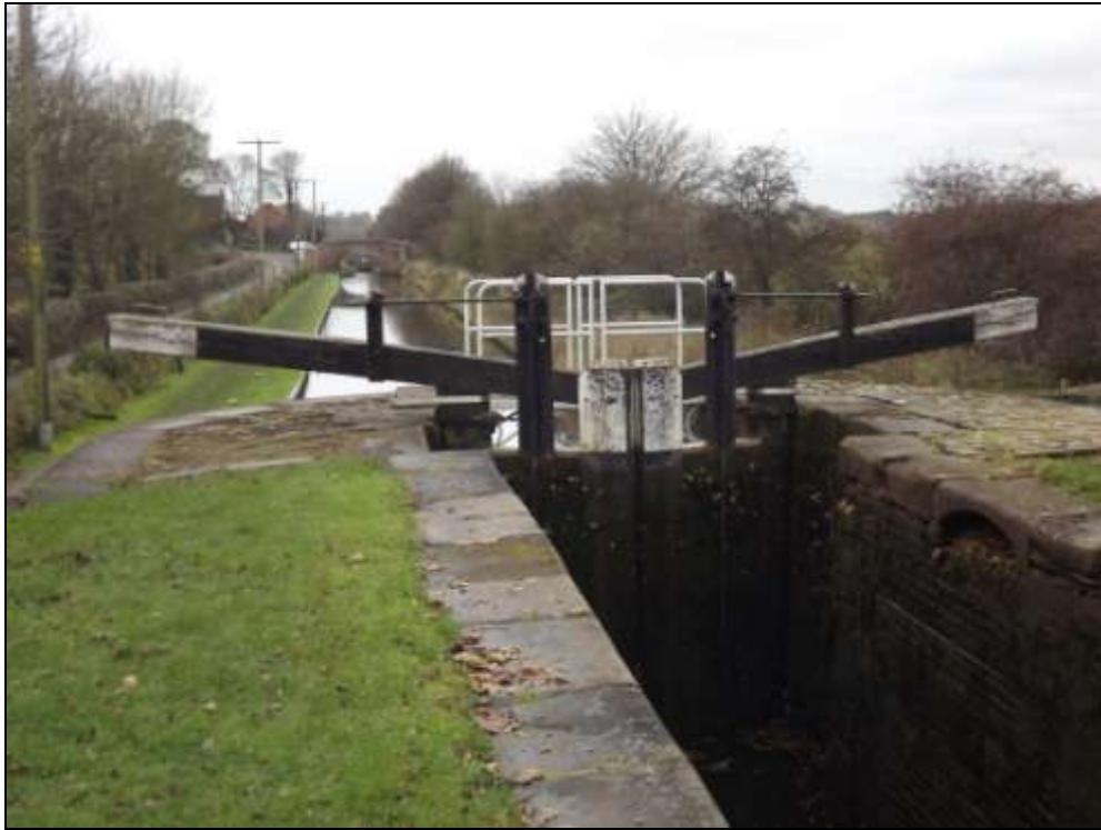
Figure 26: Sequential views towards Turnover Bridge (97)
