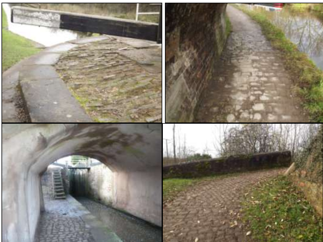
Figure 9 Surviving historic paving surfaces at Meaford locks, Barlaston, Sandon and Turnover Bridge 100
