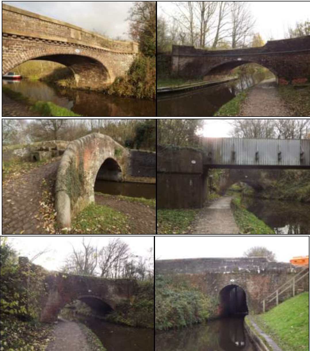
Figure 24: Bridge 102, (top left), Bridge 101 (top right), disused, with missing courses of bricks and copings. Bridge 100 (middle row, left) a turnover bridge, Bridges 99a and 99, Bridge 99, disused and heavily overgrown with vegetation. Bridge 98 (Top Lock Bridge) with damage from strike
