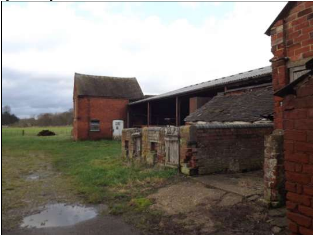
Figure 12 Pigsties at Navigation Farm
