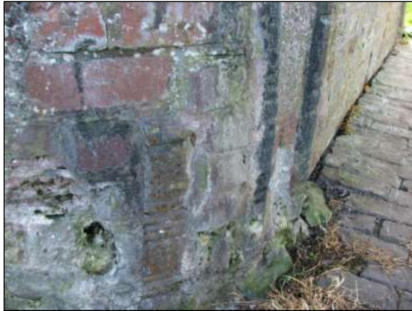
Figure 5: Grooved iron plates at Great Haywood Junction, Bridge no.109
