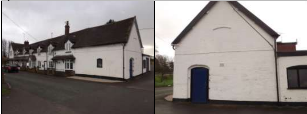
Figure 52: 1-5 Stafford Road with dormer windows and wide west gable doorway with purlins at verges
